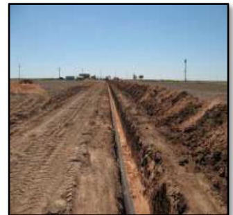
HDPE during placement in the excavation
