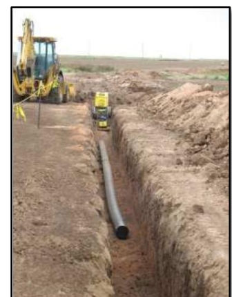
HDPE in trench. Backfilling and compaction in progress.
