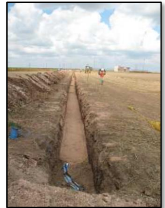
Trench during backfill operations. Utility marking tape visible in foreground.
