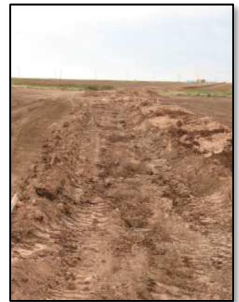
Trench during backfill and compaction activities.
