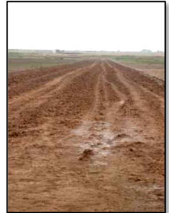
Project area during final site grading and restoration
