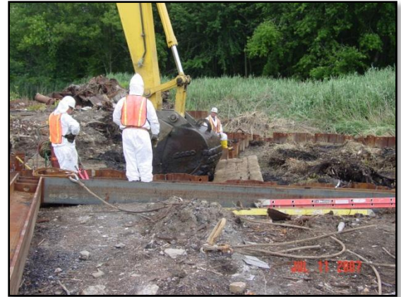
Soil Excavation at Shpack Landfill
