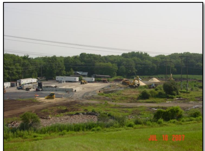
Phase II @ Shpack Landfill Remediation
