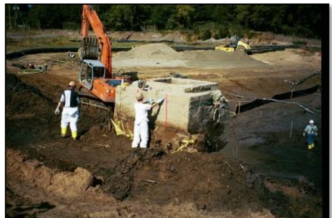
RCTs on site at Colonie FUSRAP
