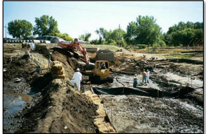
Remediation work at the Colonie FUSRAP site.
