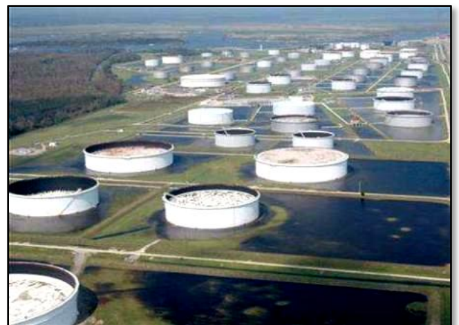
Port Arthur Tank Field
