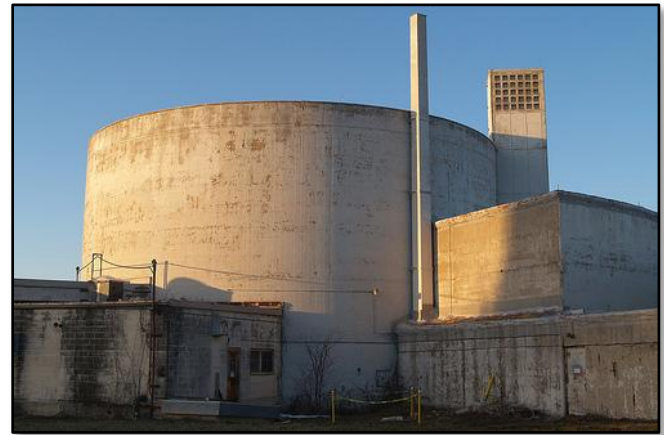
Figure 1AN L CP-5 prior to demolition in 2010; last of the Chicago Pile Reactors constructed in the 1940s
