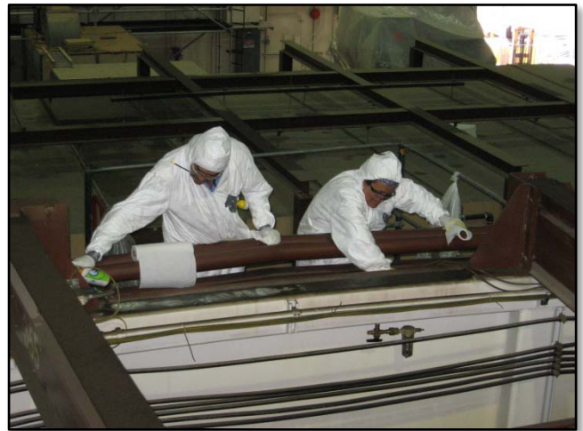
Wipe-down decontamination efforts in high bay areas of effected buildings.
