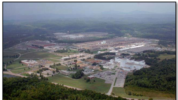
Aerial View of the East Tennessee Technology Park
